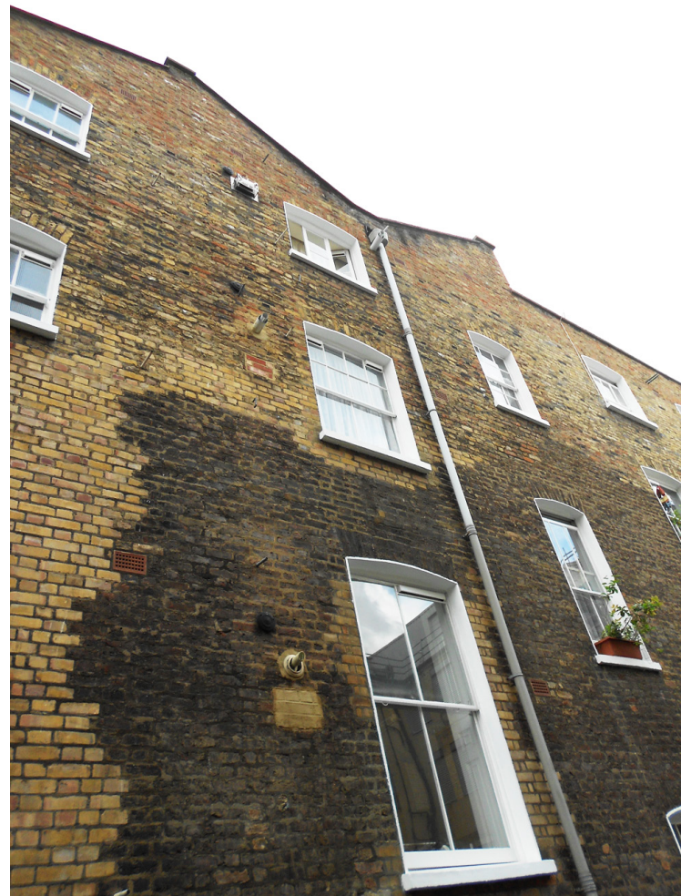
Fig.06 Image of the rear facade which clearly shows flues worked into the wall from the numerous flats. there is also new guttering and new but submissive windows in place.
