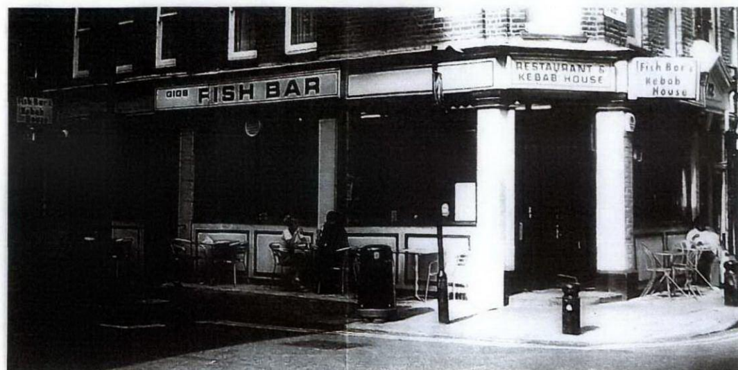
SHOP FRONT : 1950's - (PRE FIRE) 2009
