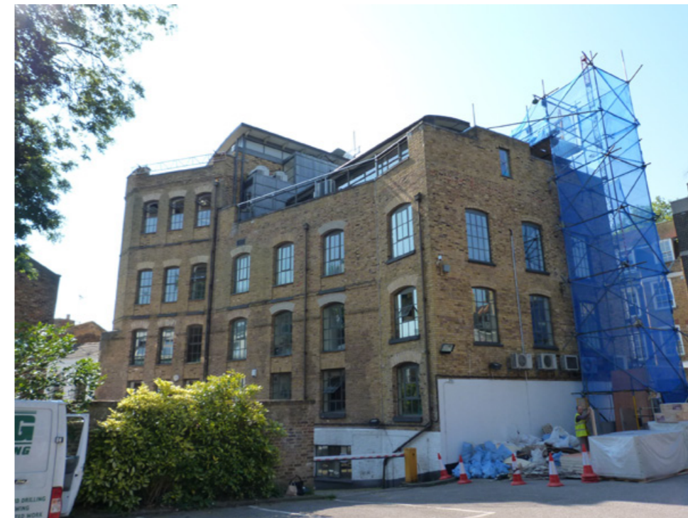
Office Building opposite carpark
