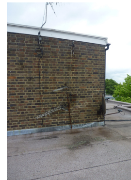
Brick structure housing lift overrun
