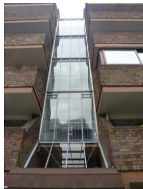
Glazing to stairwell
