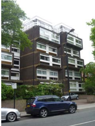
Penthouse addition at no.123 Haverstock Hill
