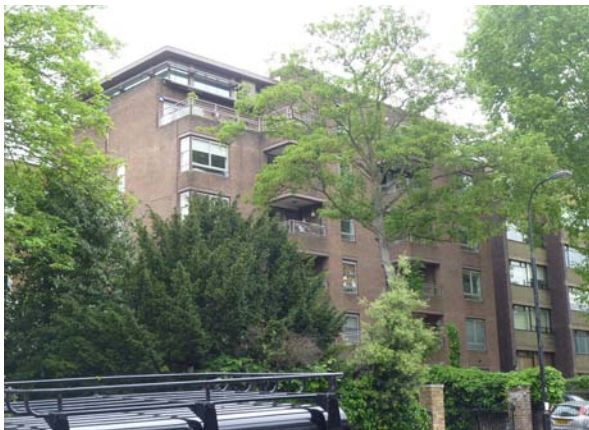
Penthouse addition at no.135 Haverstock Hill
