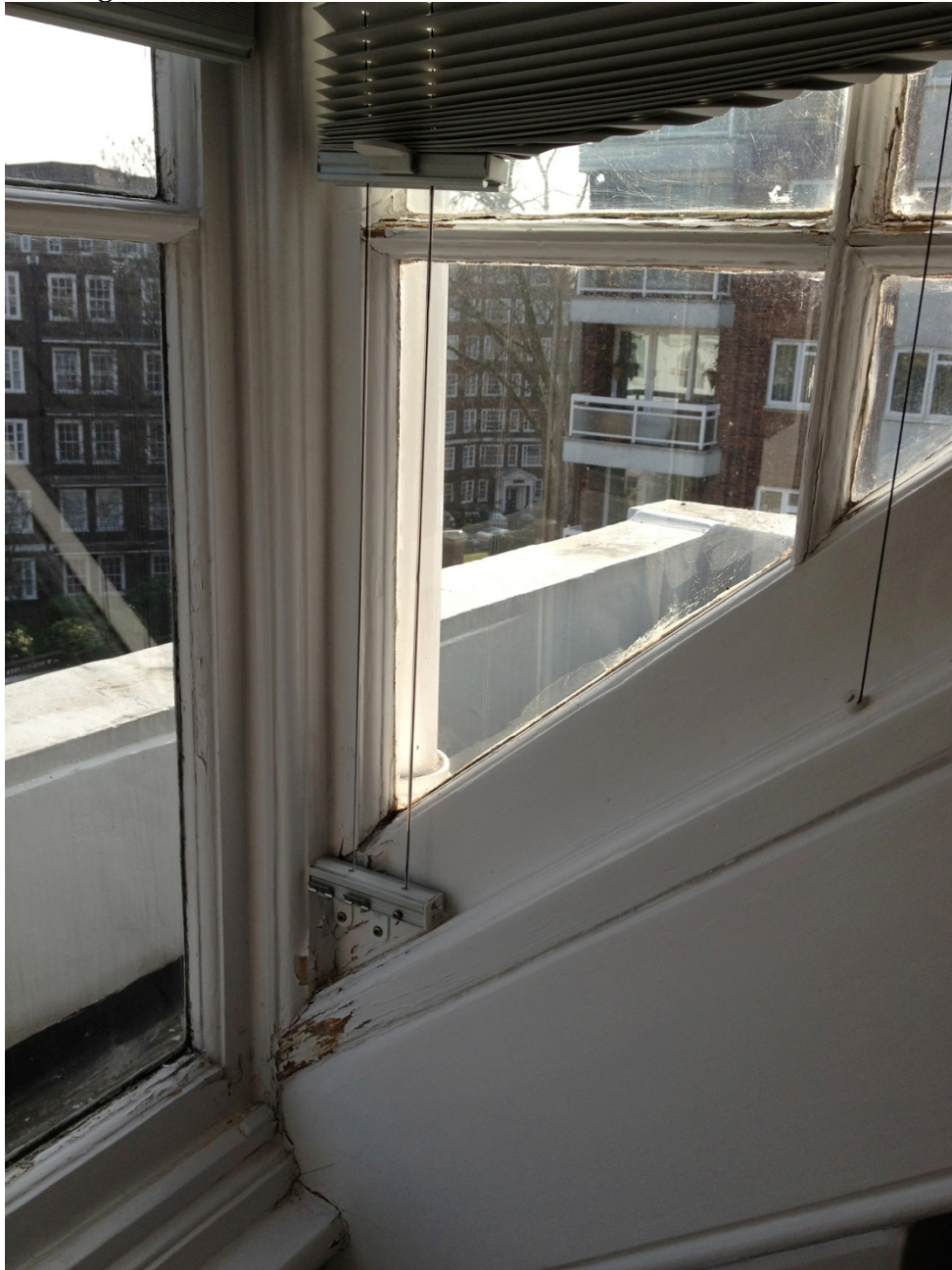
13 Eton Villas Existing Windows
