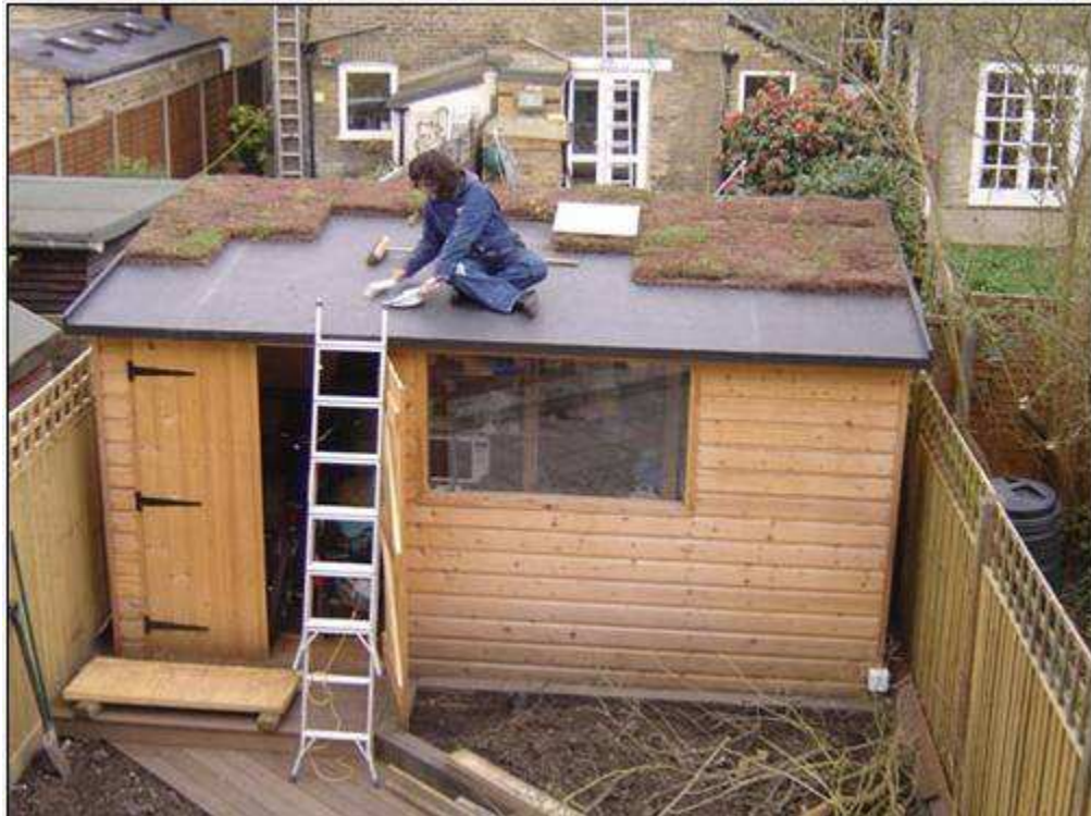
P13. Lay Sedum Tiles, side by side
