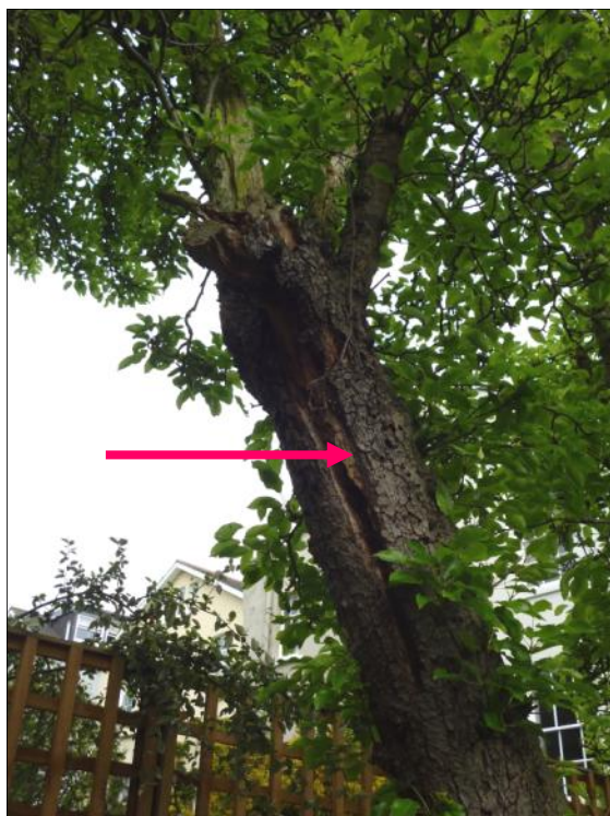
5. Photo of crack in the main branch of T4
