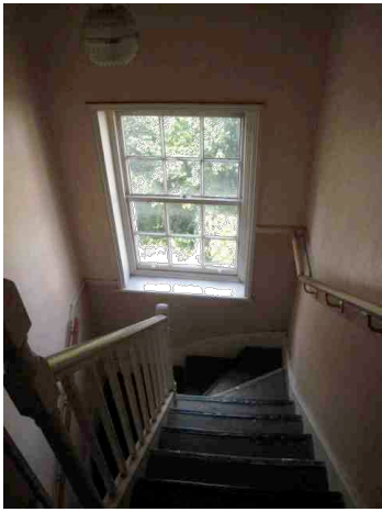
non-original handrails to be removed
