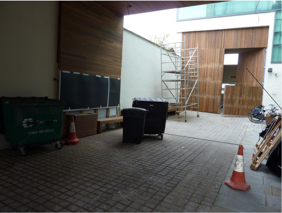
View from covered parking area towards existing Bin Store enclosure, (see plan adjacent)
