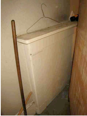
blocked fireplace (damaged mouldings)
