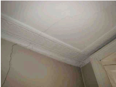
vertical crack (extends to ceiling)
