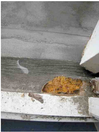
defective cill to roof terrace doors
