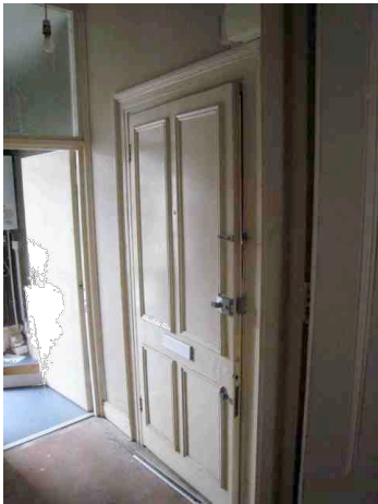
original door with fireproofed panels and raised mouldings
