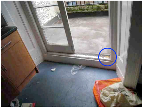
non-original roof terrace doors(defective cill circled)
