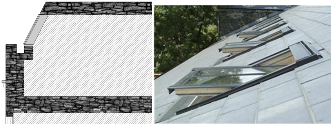
Sloped Velux/conservation window alternative
