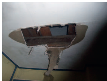
Large area if ceiling missing, areas of bulging, loose or blown plaster
