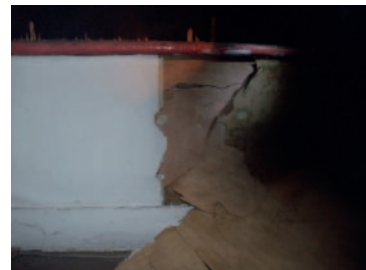
under window damp areas, painted, paper, boarded - falling away
