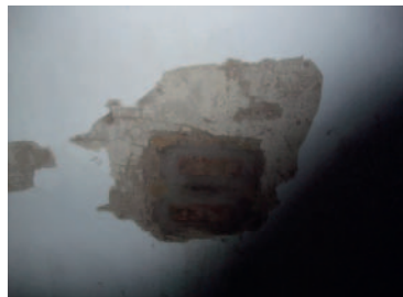
painted, areas of plaster blown, internal brick
