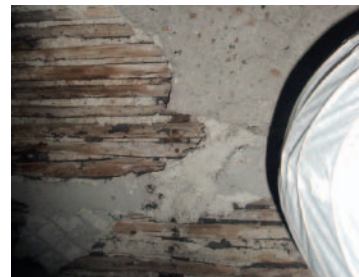
Large area if ceiling missing, remaining loose
