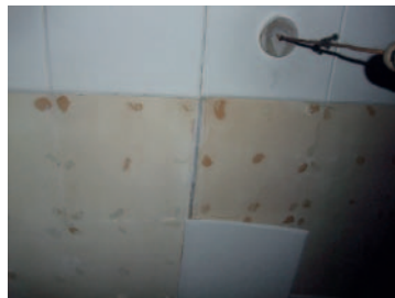
tile covered ceiling, papered ceiling, signs of movement - loose areas of plaster
