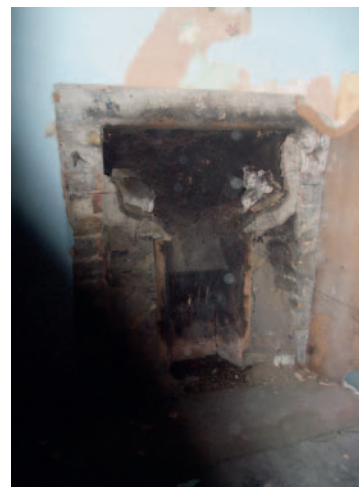
exposed brickwork where fireplace taken away
