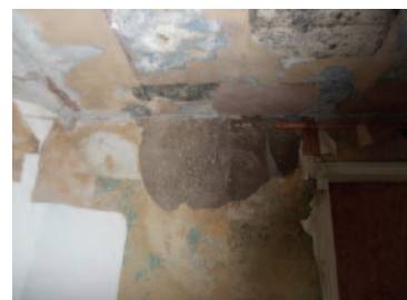
4th floor, serious damp, papers and paints falling away, plaster wet
