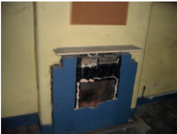
ROOM S15 FIREPLACE S15 MISSING - REPLACE WITH SALVAGE
