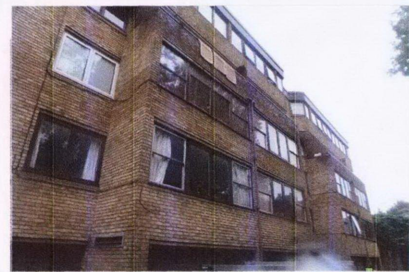
Photograph illustrating the mixture of existing window frame finishes
