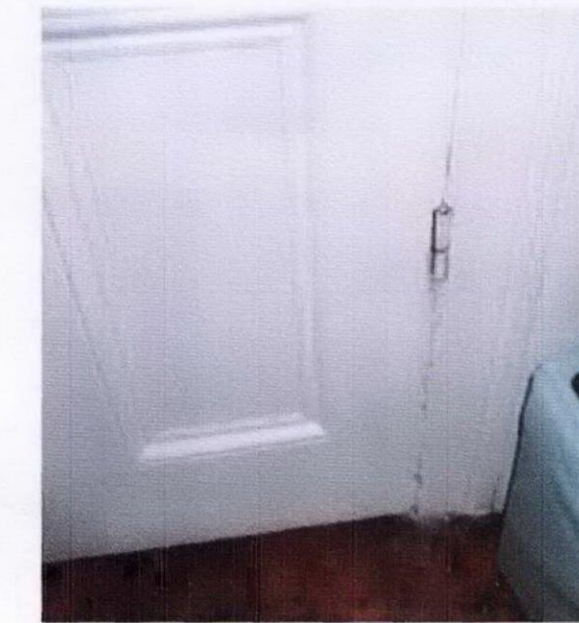
PHOTOGRAPH OF EXISTING DOOR DETAIL WITH MOULDINGS
