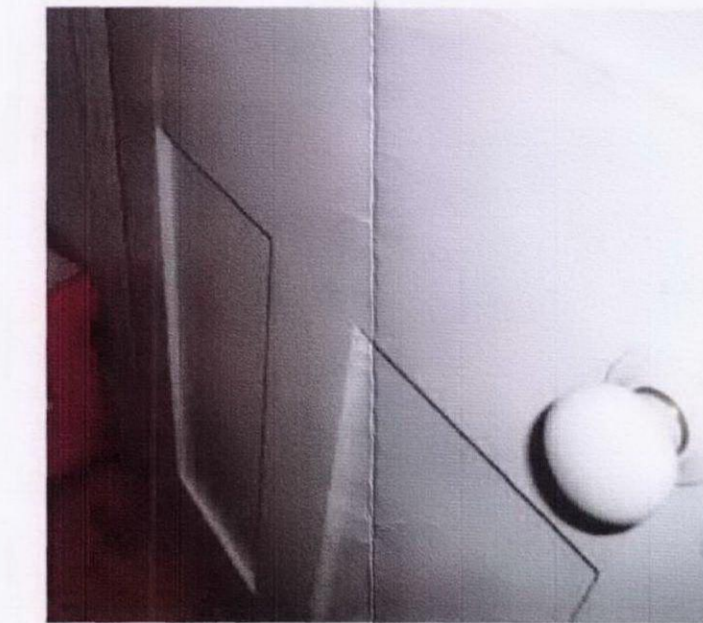
PHOTOGRAPH OF EXISTING DOOR DETAIL WITHOUT MOULDINGS
