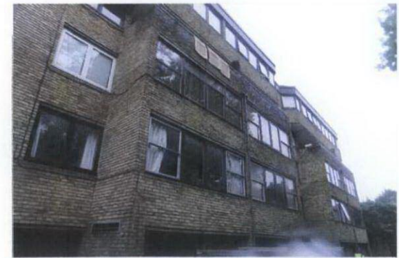
Photograph illustrating the mixture of existing window frame finishes
