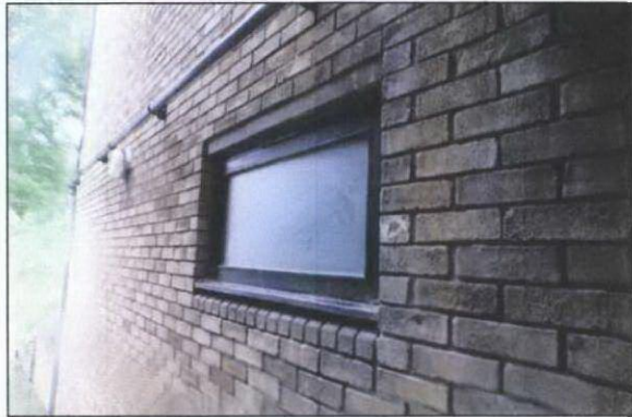
Photograph illustrating relationship of existing window cill to existing chamfered brickwork
