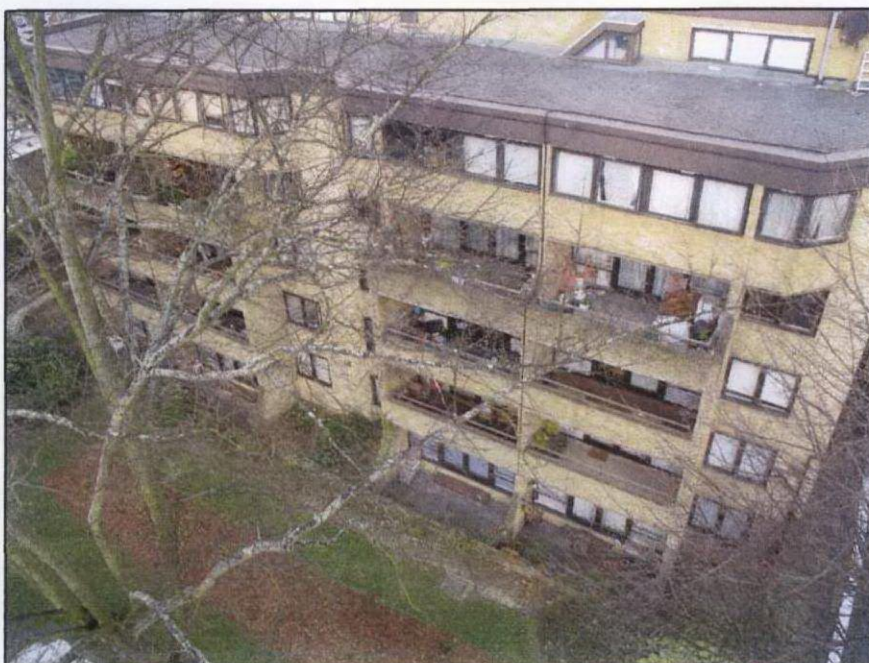
Figure 1. Front Elevation, 15 Belsize Av.
