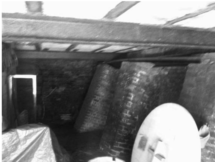
Plate 5 - Revetments in retaining wall in lower floor of structure.
