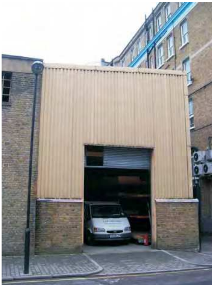
Plate 7: Structure on the site of the former Red Lion Public House
