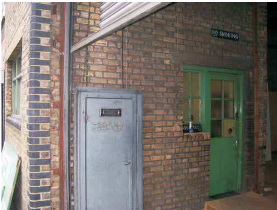
Plate 2: Office room at the front of the site
