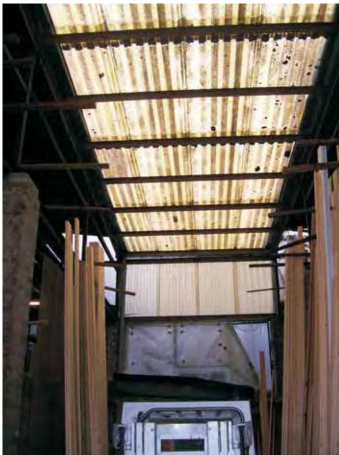
Plate 5: Temporary roofing on the centre of the site
