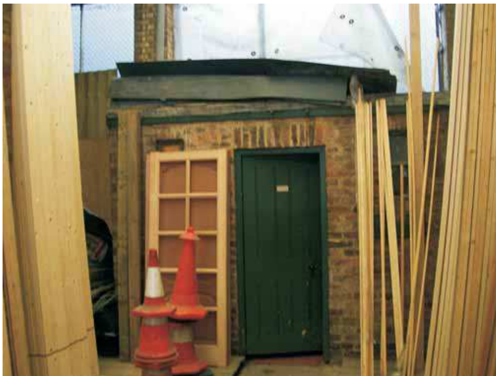
Plate 3: Bathroom block toward the rear of the site
