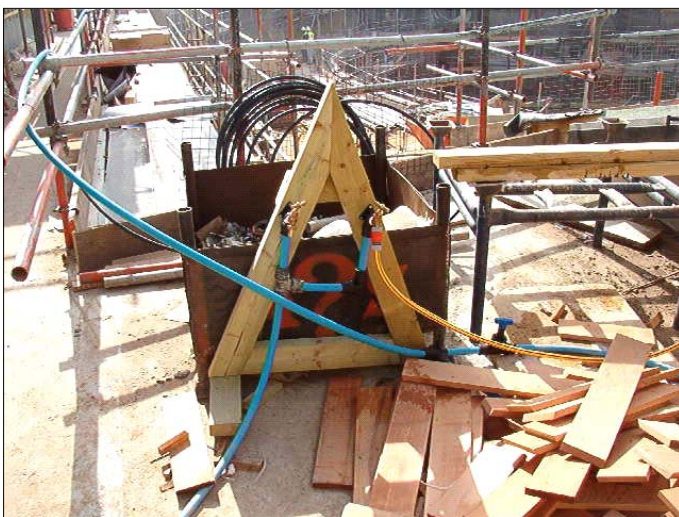
An example of a temporary watering system rigged up on site to provide an adequate mains watering feed to different roof areas.
