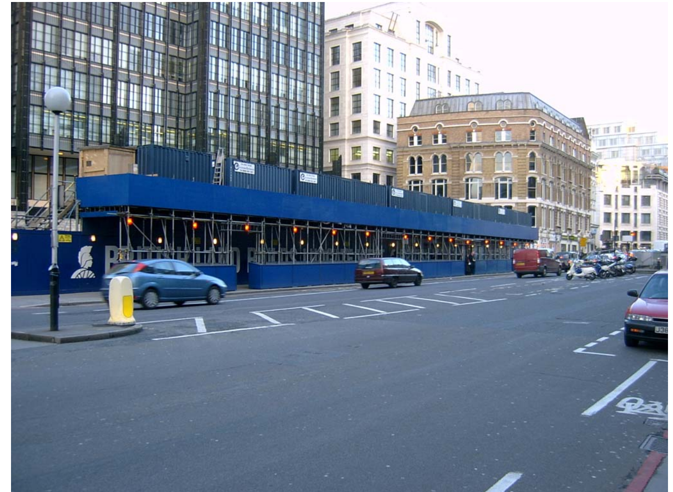
Figure 4 Example of protective gantry
