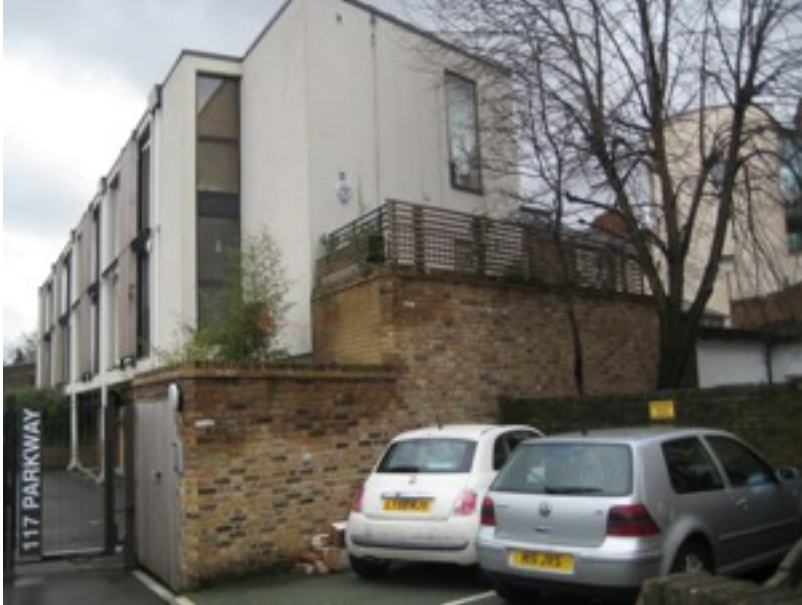
View of House 1, existing terrace. Photograph taken in winter showing the outlines of the Lime tree in the adjoining garden of 121 parkway
