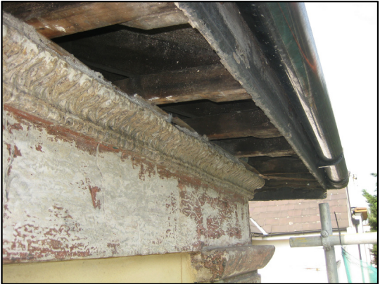
Failure of the lath & plaster eaves resulted in some water ingress that lead to some minor damage to the roof structure
