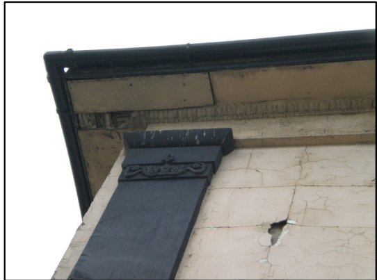
The damage lath and plaster used at eaves level was extensively damaged wherever it was used.
