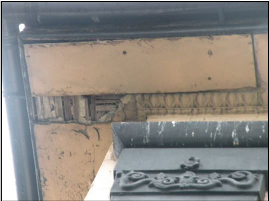
Close up of the damaged lath and plaster, and the plywood board repairs.
