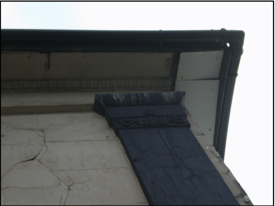
Failure of the original lath and plaster lead to the use of plywood boards to cover the exposed roof structure
