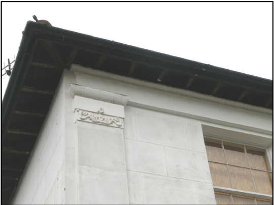
Current condition following removal of decayed materials
