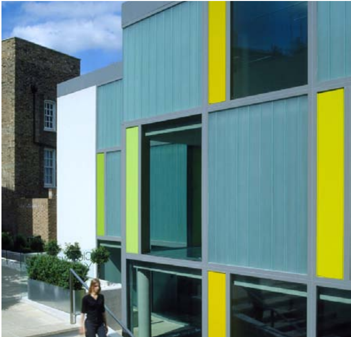
AHMM - Clearwater Yard. Curtain wall with cast glass channels and opening opaque panels.
