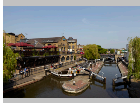
2 | Camden Lock Footbridge
