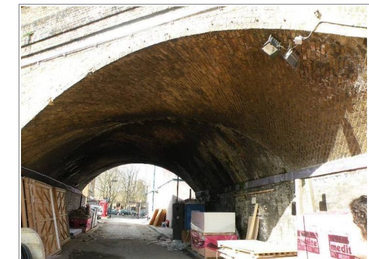
Fig. 19 Skewed brickwork arches within the subject site.
