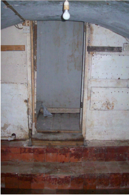
Photo 25 – Western vault with metal sheet lining (3.7.3)
