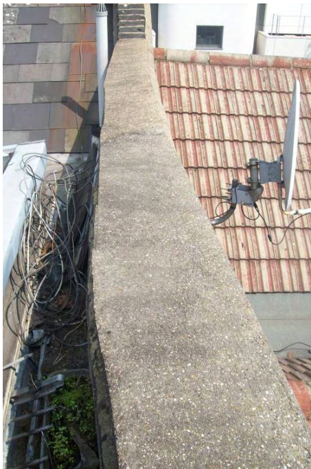
Photo 19 – Deflection to south parapet (3.3.12)
