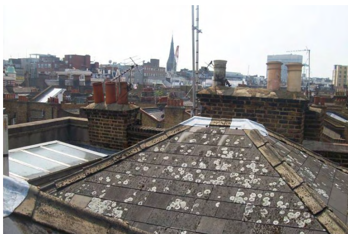
Photo 3 – Pitched roofs showing replacement artificial Slates and repairs (3.1.3)
