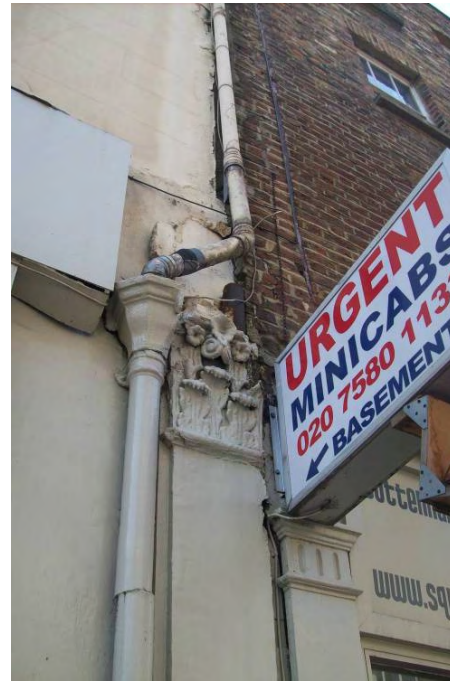
Photo 12 – Defective rainwater goods at Tottenham Street elevation (3.2.4)
