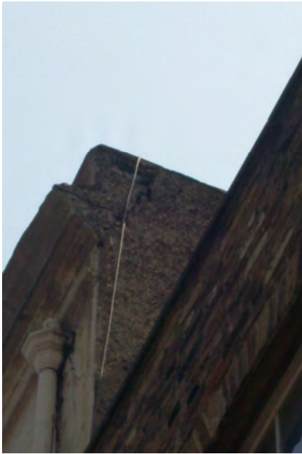
Photo 17 – Fracture in corner of parapet on Tottenham Street elevation (3.3.8)
