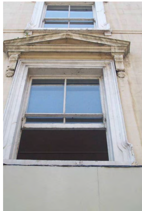
Photo 20 – Typical double hung vertical sash window (3.4.1)
