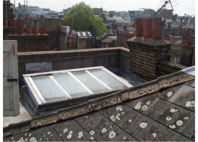
Photo 6 – Defective laylight (3.1.10)
