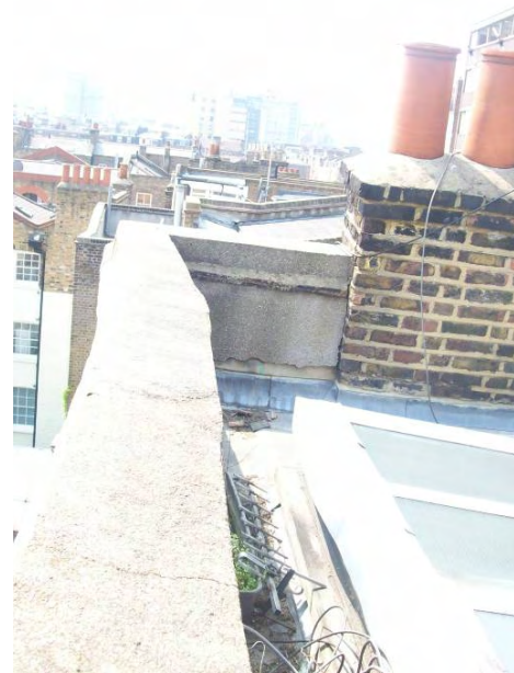
Photo 8 – Leaning brick stack and deflecting parapet on south west corner (3.1.14)
