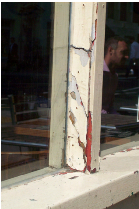
Photo 21 – Piece in repairs to shop front joinery (3.4.8)
