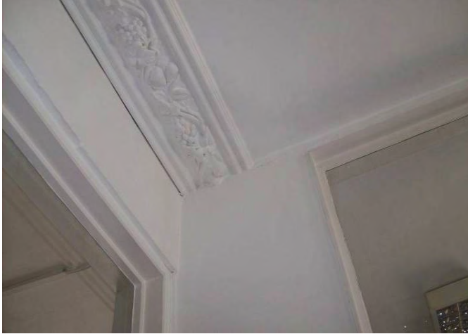
Photo 37 – Detail of moulded cornice on first floor (3.10.10)
