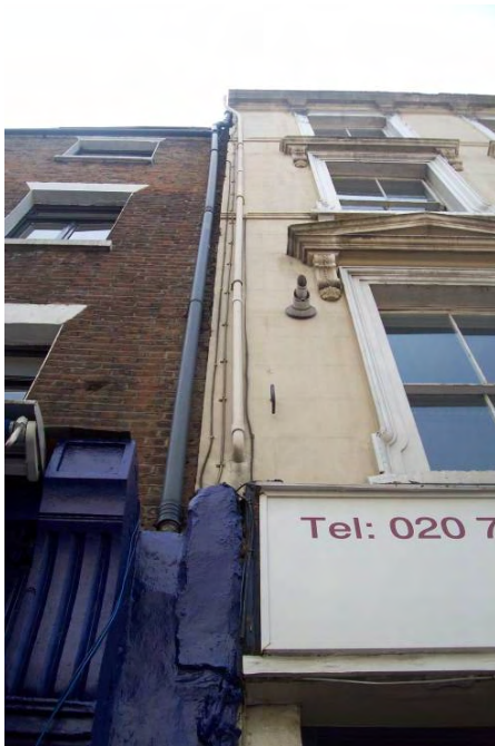
Photo 13 – Rainwater outlet on south side of Charlotte Street elevation (3.2.5)
