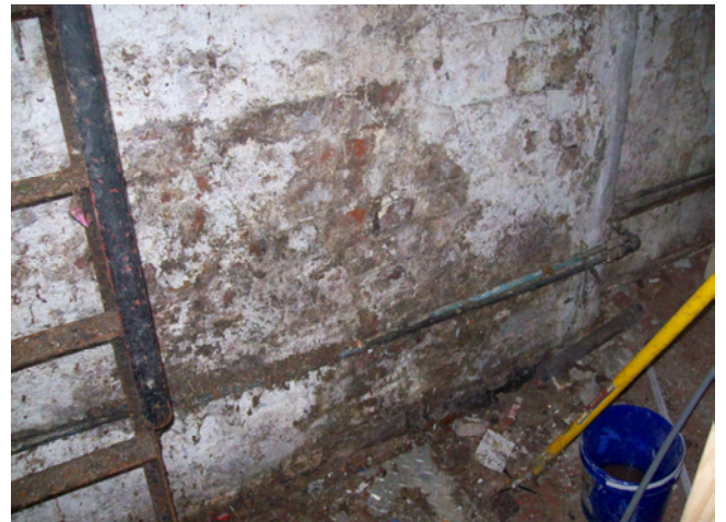
Photo 28 – Damp to external basement wall on east side (3.7.8)
