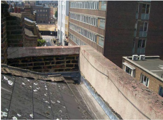
Photo 5 – Valley gutter and outlet at north west corner (3.1.8)
