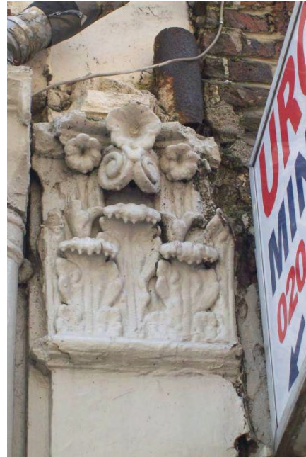
Photo 14 – Damaged detail of capital on Tottenham Street elevation (3.3.4)
