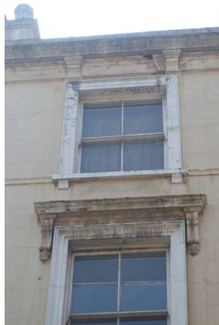
Photo 16 – Vertical fracture on upper floors on east side of Tottenham Street (3.3.8)
