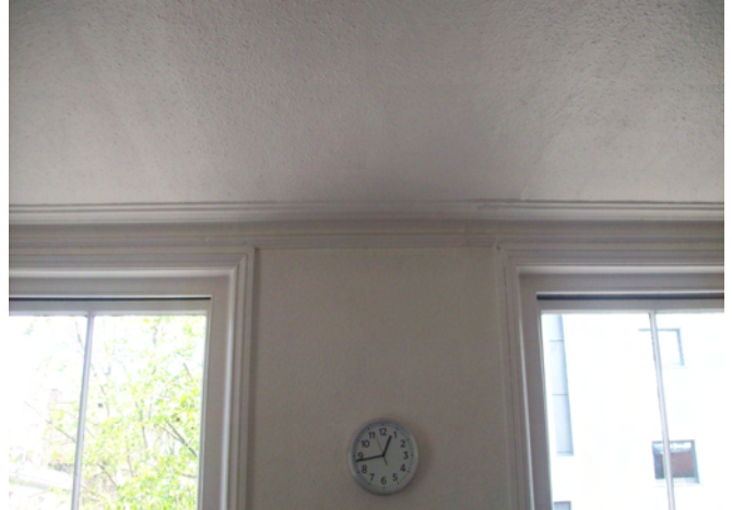
Photo 38 – Movement at wall/ceiling junction on second floor (east wall) (3.11.7)
