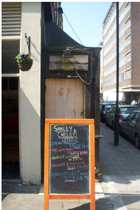
Photo 15 – Poorly built access structure to basement (3.3.5)
