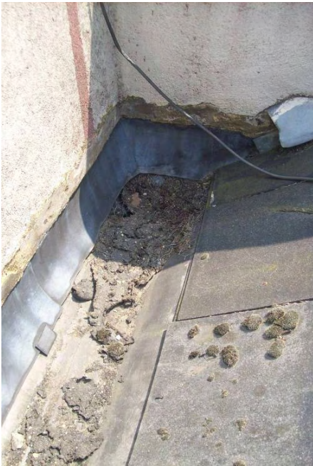
Photo 11 – Roof outlets prone to blocking (3.2.2)
