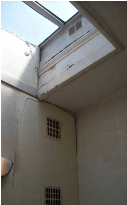
Photo 35 – Defective laylight (3.9.8)
