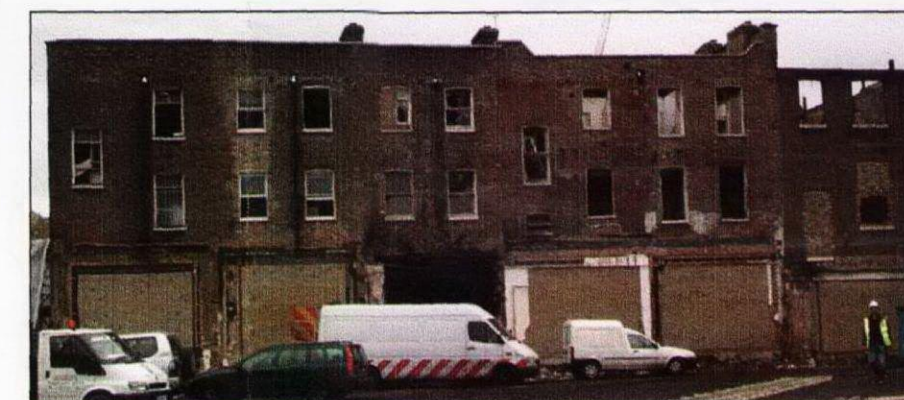
IMAGES OF EXISTING BUILDING FAÇADE
