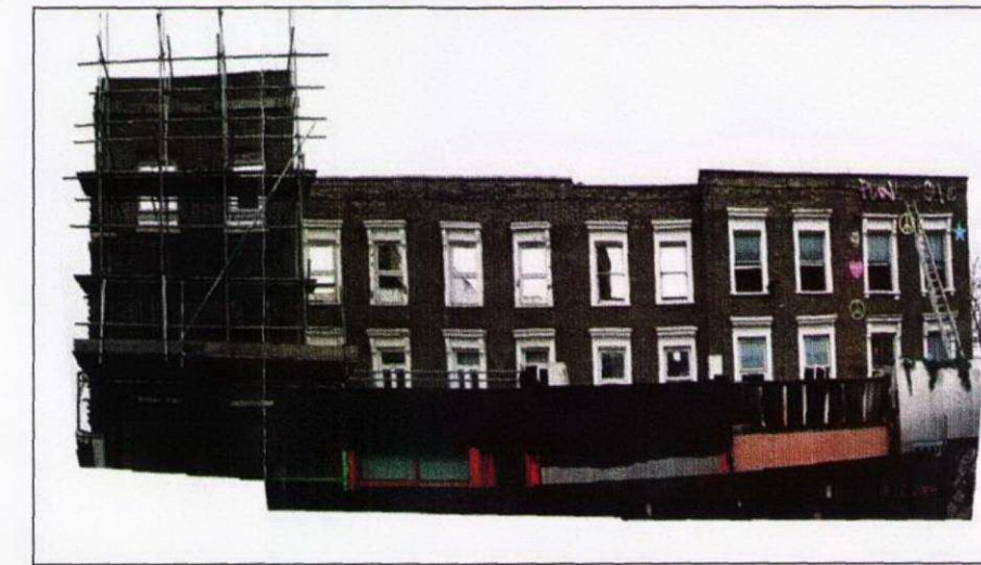
IMAGES OF EXISTING BUILDING FAÇADE
