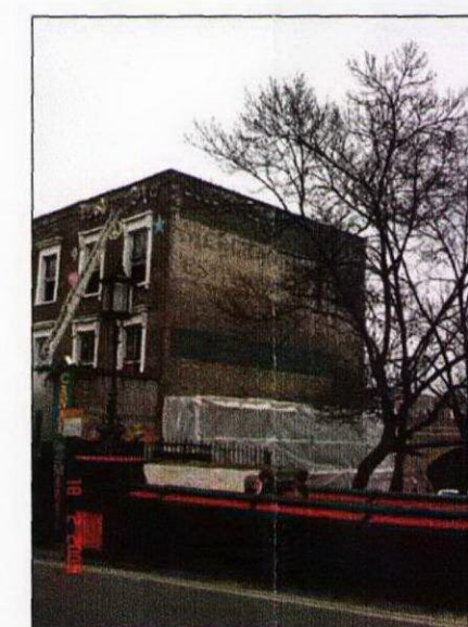
IMAGES OF EXISTING BUILDING FAÇADE
