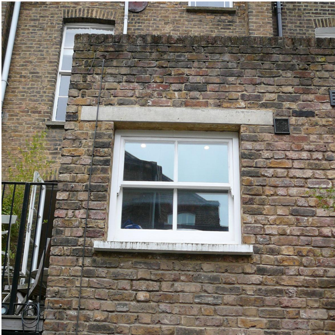
Figure 3. Horizontally proportioned window in extension with concrete cill and lintel to be replaced
