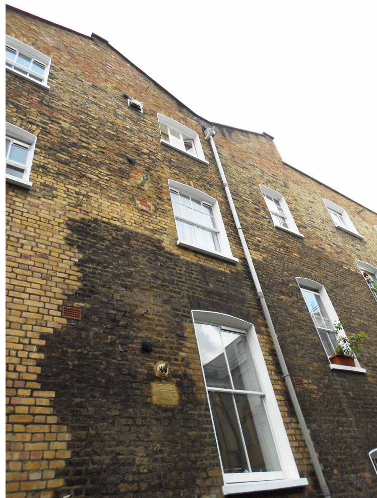
Fig.06 Image of the rear facade which clearly shows flues worked into the wall from the numerous flats. there is also new guttering and new but submissive windows in place. We intend to preserve the original windows that are currently in situ.
