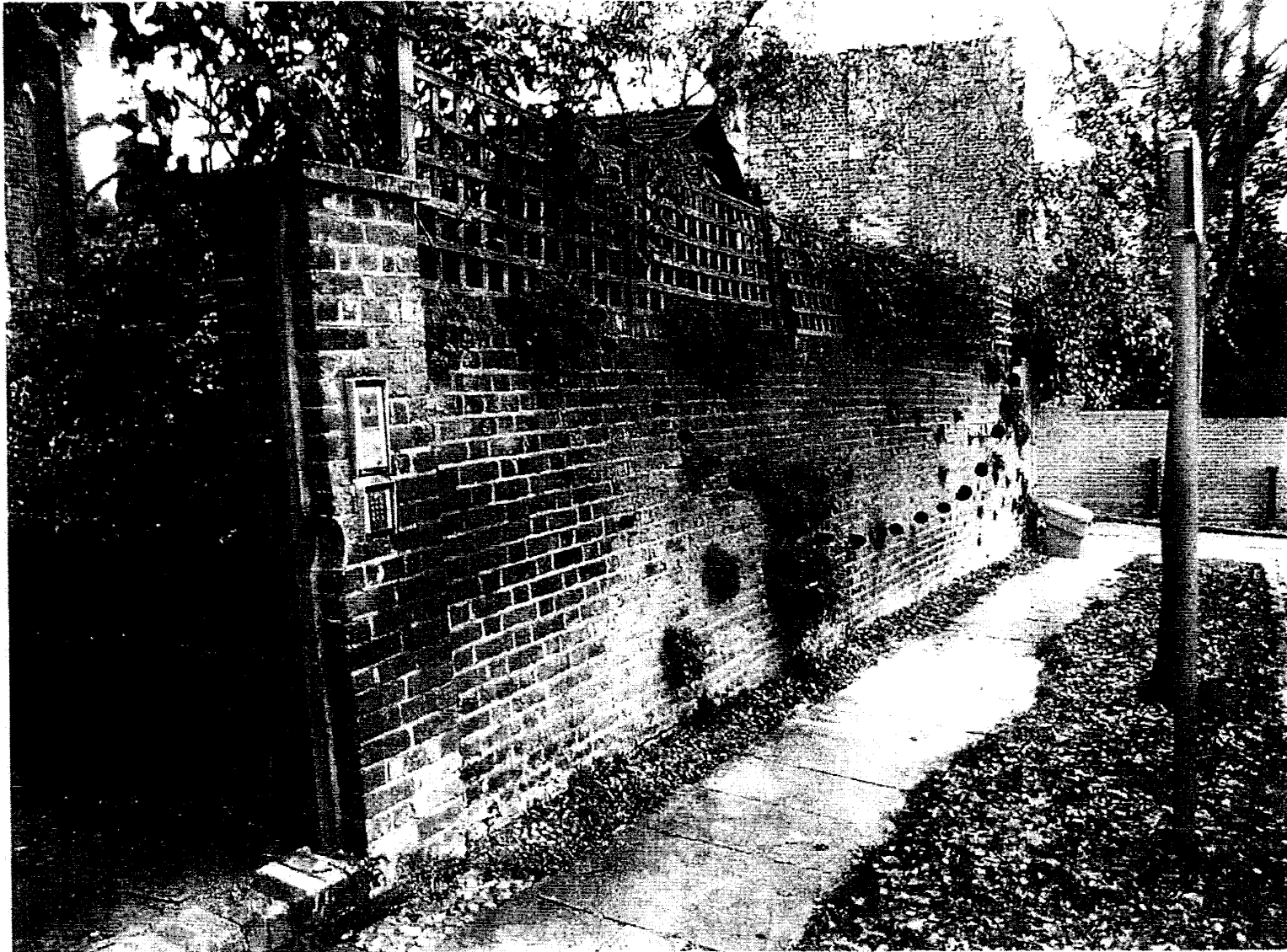
D3878/002 - Photo illustration of wall to be re-built. 13/08/12
