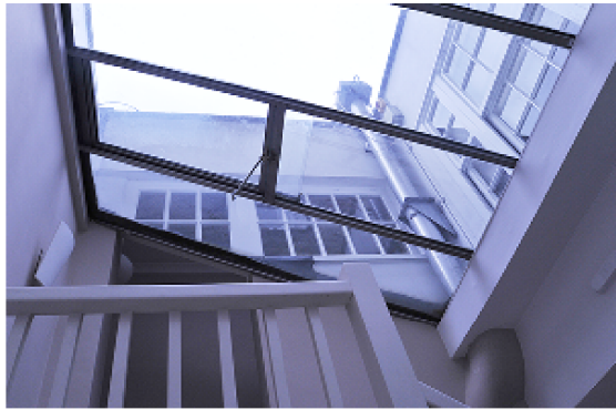
IMAGE OF EXISTING SINGLE GLAZED ROOF LIGHT LOOKING UP FROM GROUND FLOOR
