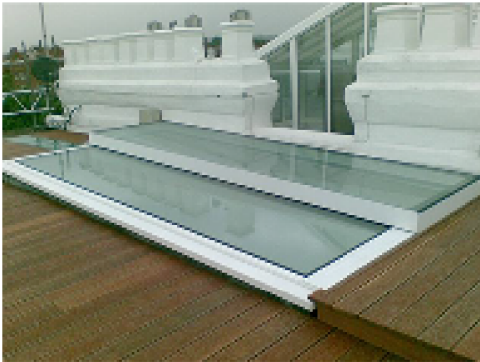
SLIDE OPENING DOUBLE GLAZED AUTOMATED ROOF LIGHT IN POWER COATED STEEL FRAME
