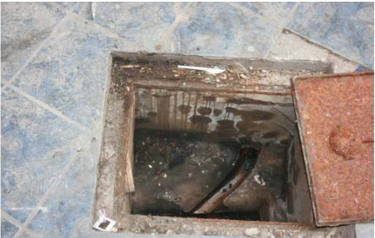
Photo 6 Detail of manhole in rear yard 0.8m deep with outlet draining to front of Cleveland Street
