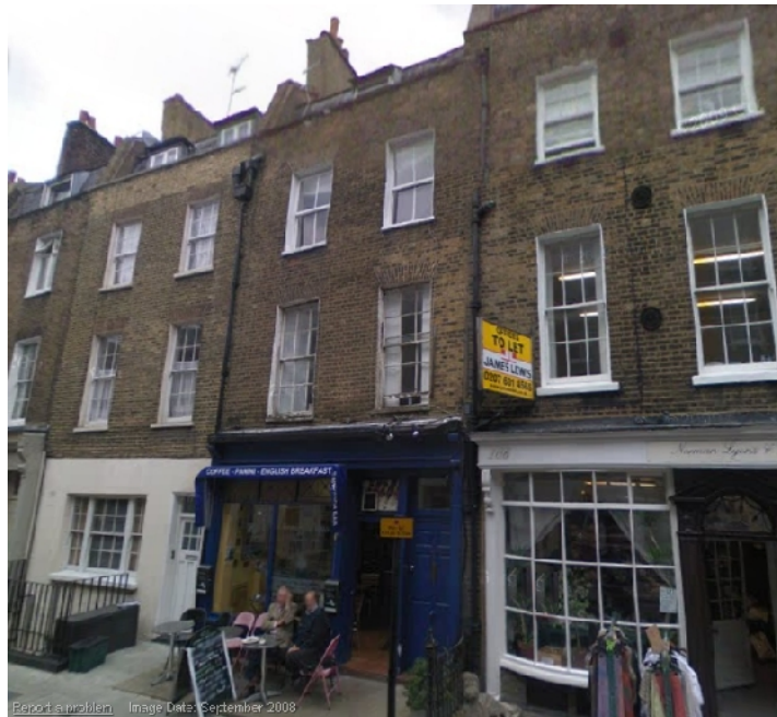
Figure 1 Front Elevation of 108 Cleveland St, seen in centre of the image
