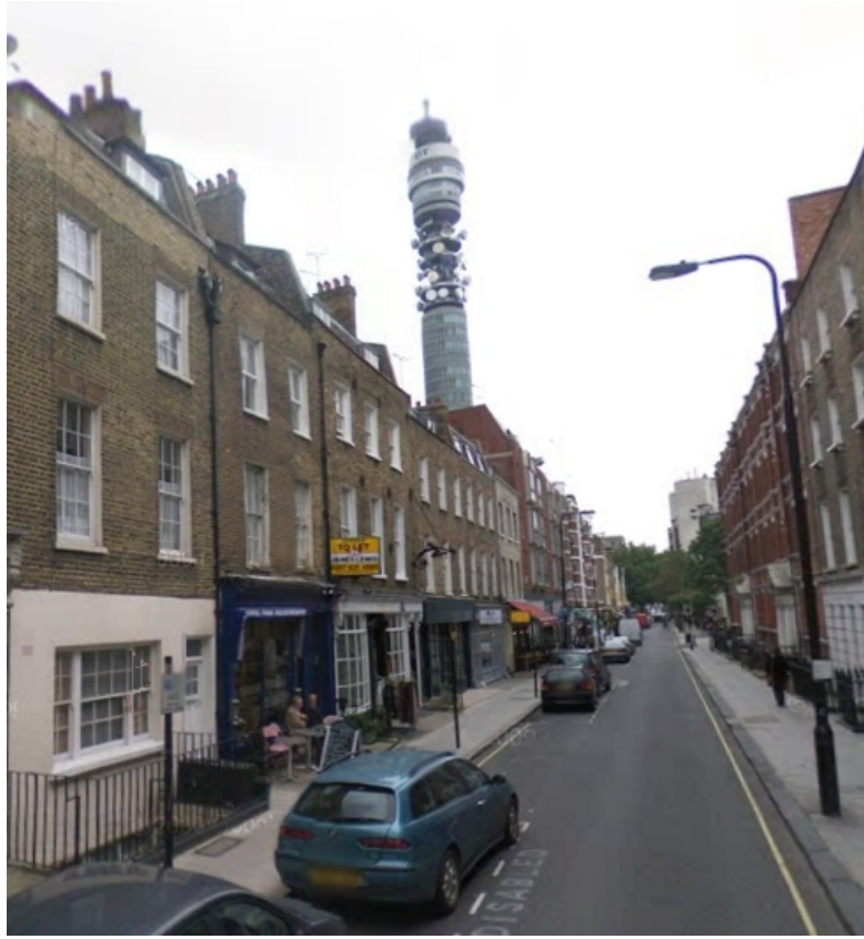
Figure 2 existing street scene of Cleveland Street
