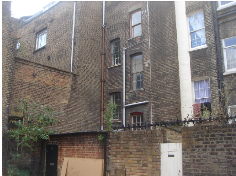
Figure 3 Rear Elevation of No 108 Cleveland Street
