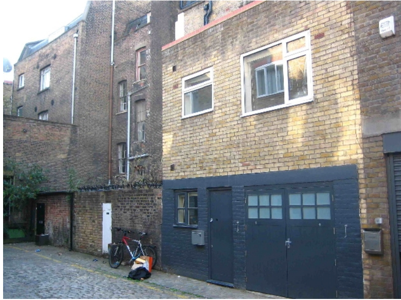
Figure 4 Rear elevations of No 108-112 Cleveland Street, forming Warren Mews
