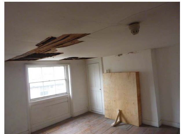
Room 3.02 Showing 1980's plaster ceiling
