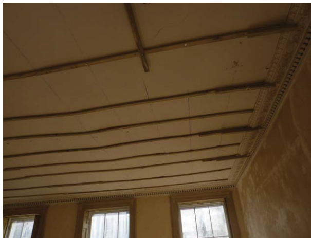
Room 1.01 Supporting cracked ceiling and cornices
