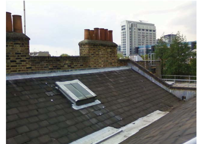
Repair required to existing roof including creating access hatch through existing rooflight
