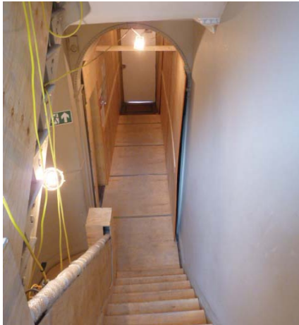
Room G.03 Protection of stair, wall panelling and front door
