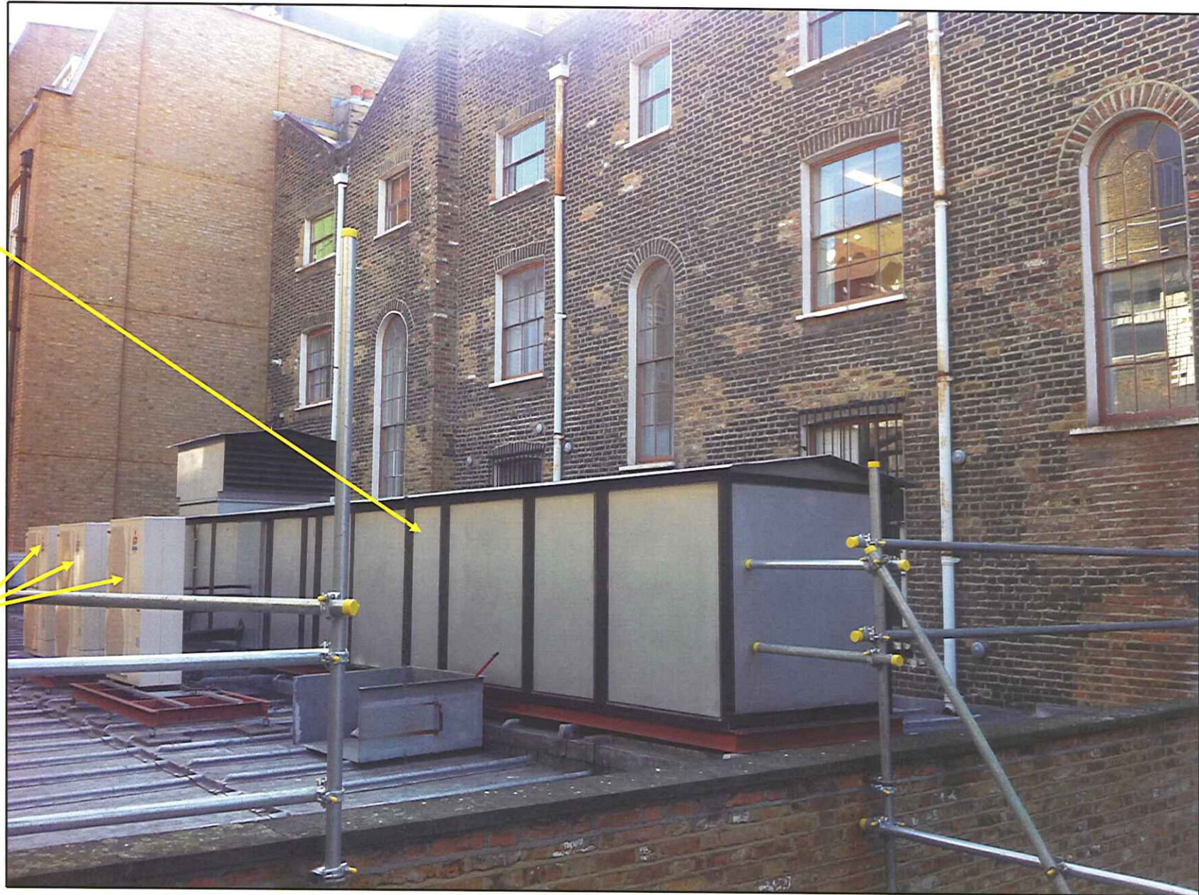
PHOTO C: Rear façade of Venezuela Consulate building with Air Handling unit and Condenser on first floor roof.
