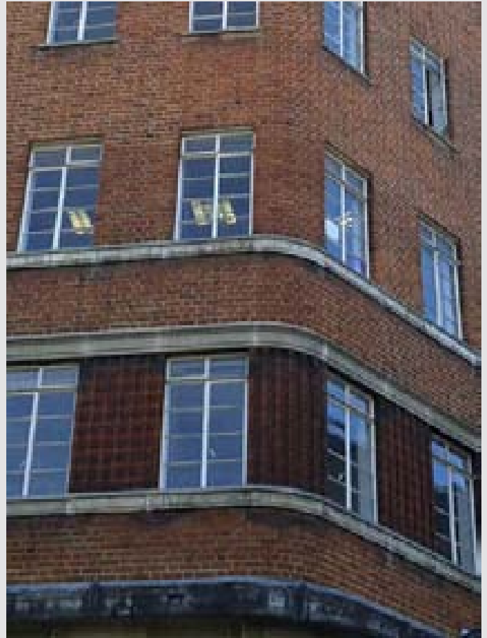
Brickwork - in need of repair
