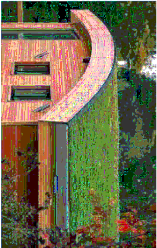
Example of Sedum Green Roof used with timber cladding.
