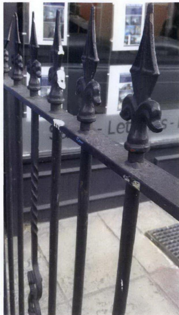
3A View of Existing Railing
