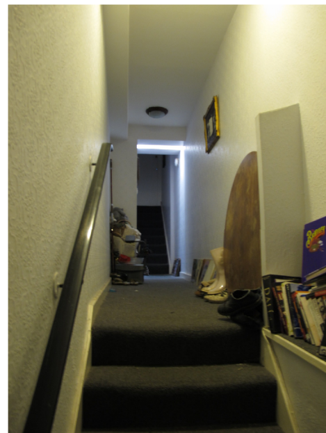
11 First Floor Staircase (No daylight)
