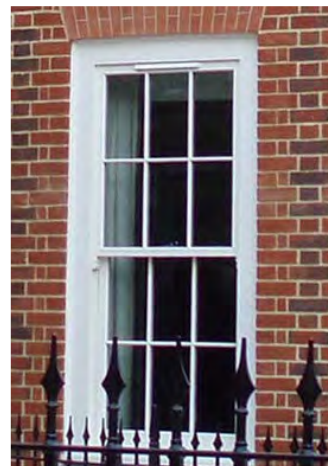
Ground floor 6/6 sash window
