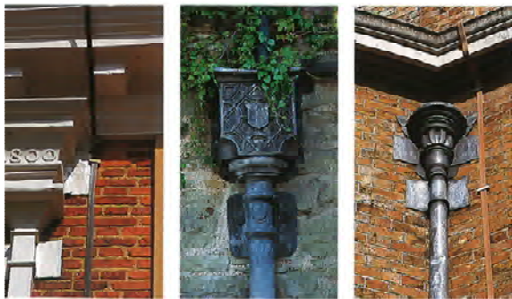
Georgian cast iron headers and down pipes
