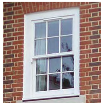
First floor 6/6 sash window
