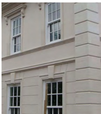
Stacked quoins in stone/stucco
