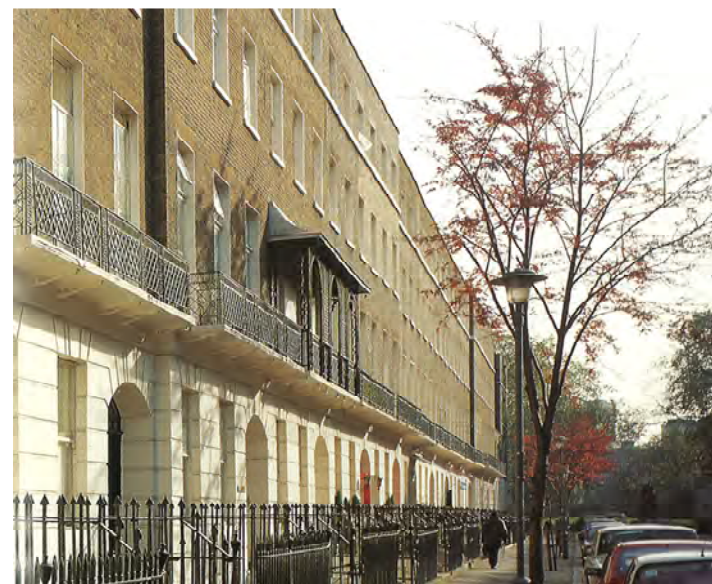
Ground floor banding in stucco to imply stone, brick above
