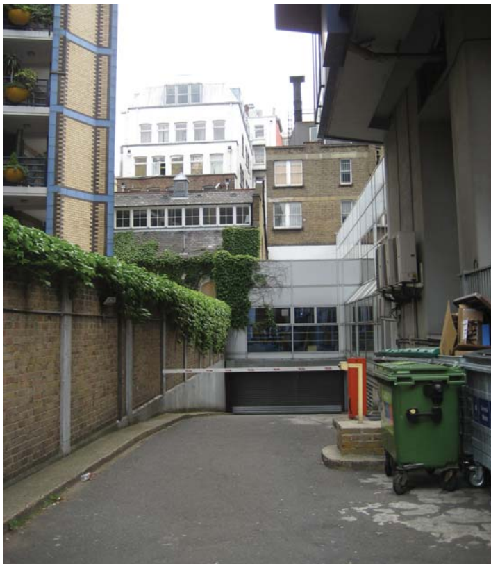
Photo showing the rear of Craven House as viewed from Newton Street. The proposals will not be visible from either Newton Street or Kingsway.
