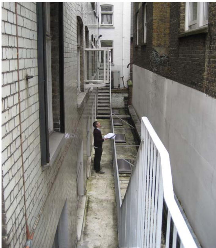
Photo showing the existing mezzanine roof area. The proposed UKPN grille will be installed at the far end underneath the first floor window. The existing stair shown at the far end has already been removed.
