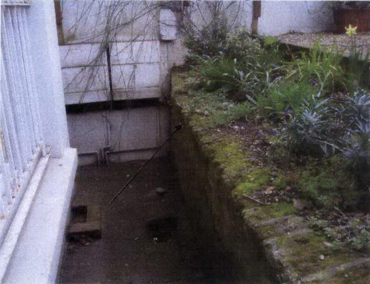
View of movement to front retaining wall
