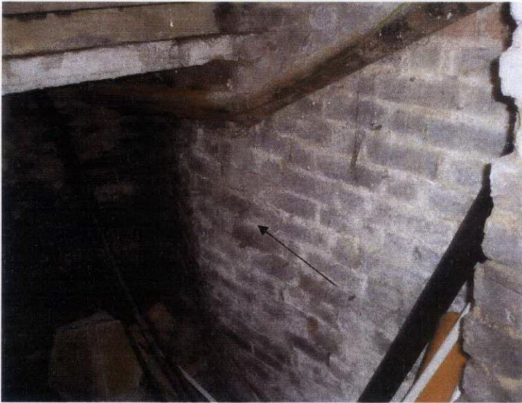
View of bulging wall in understeps storage area
