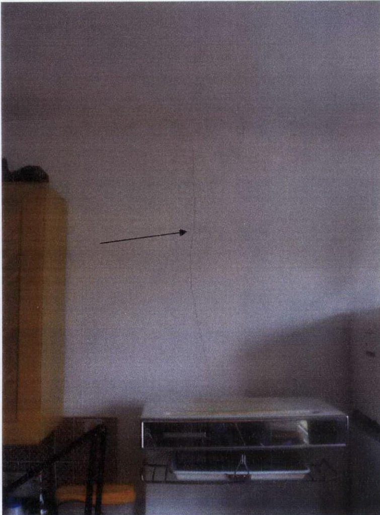
Cracking to right hand party wall in 2nd floor flat lounge / kitchen
