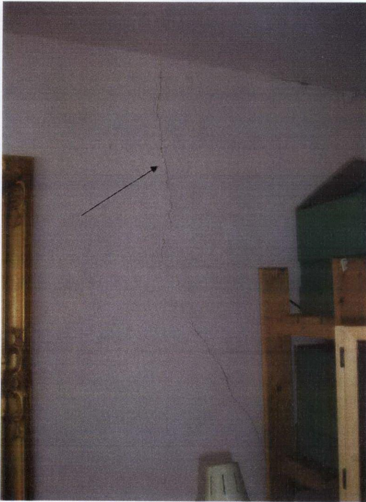
Cracking to left hand party wall in 2nd floor flat lounge / kitchen
