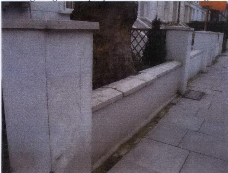
View of tree growing against and pushing front boundary wall
