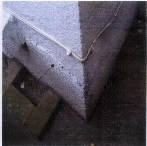
Cracking to bay
