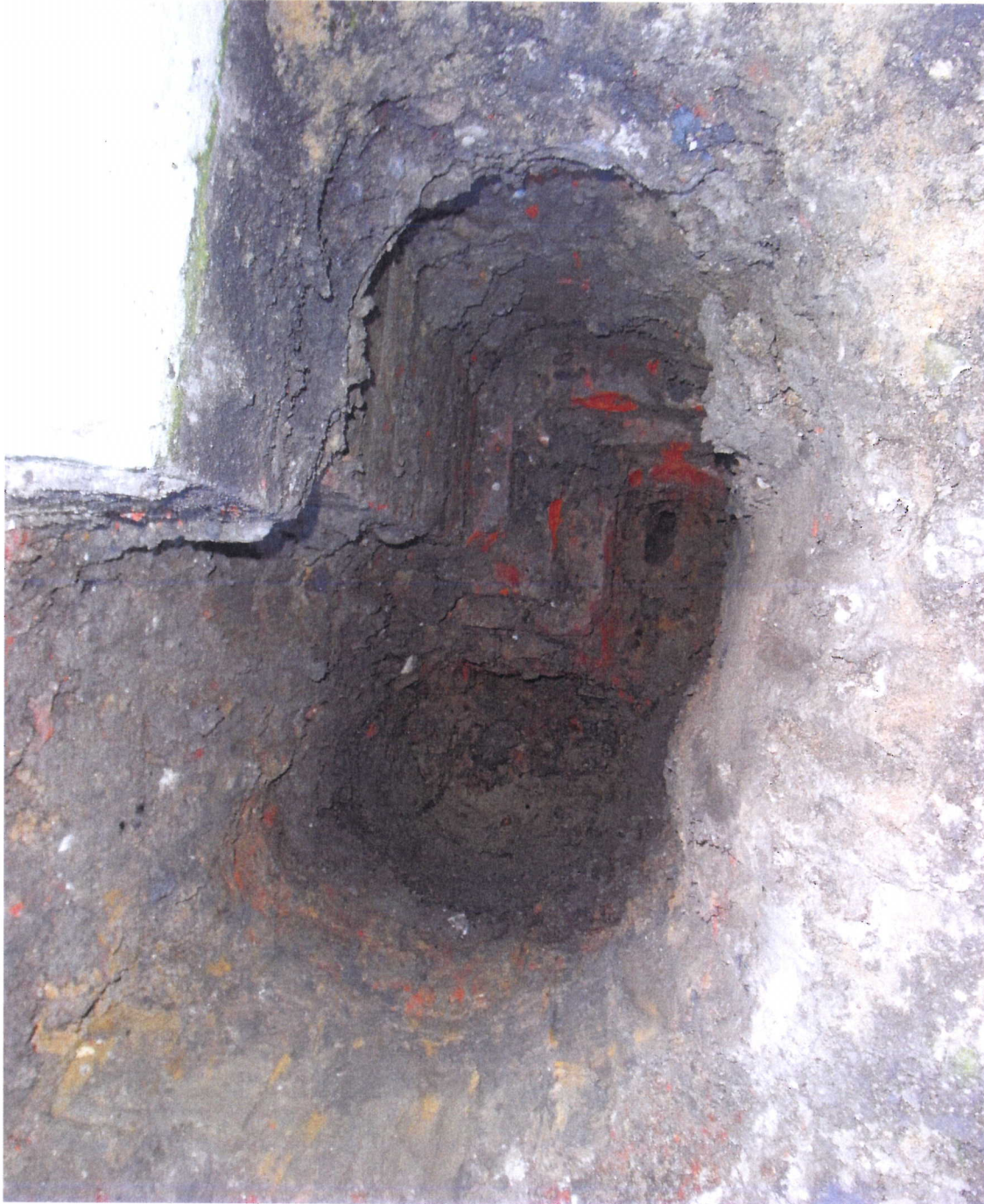
View of the footings encountered in Trial Pit No 1, looking south (16/11/2010)
