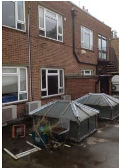
04. Rear Elevation and roof of Ground Floor, facing South
