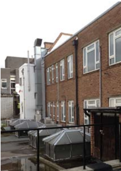
03. Rear Elevation and roof of Ground Floor, facing North
