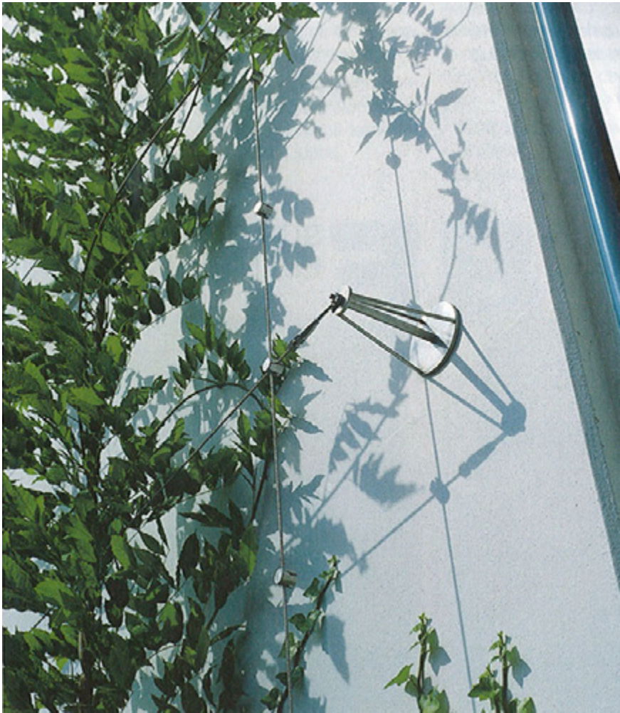
Climbing wire system to retaining wall
