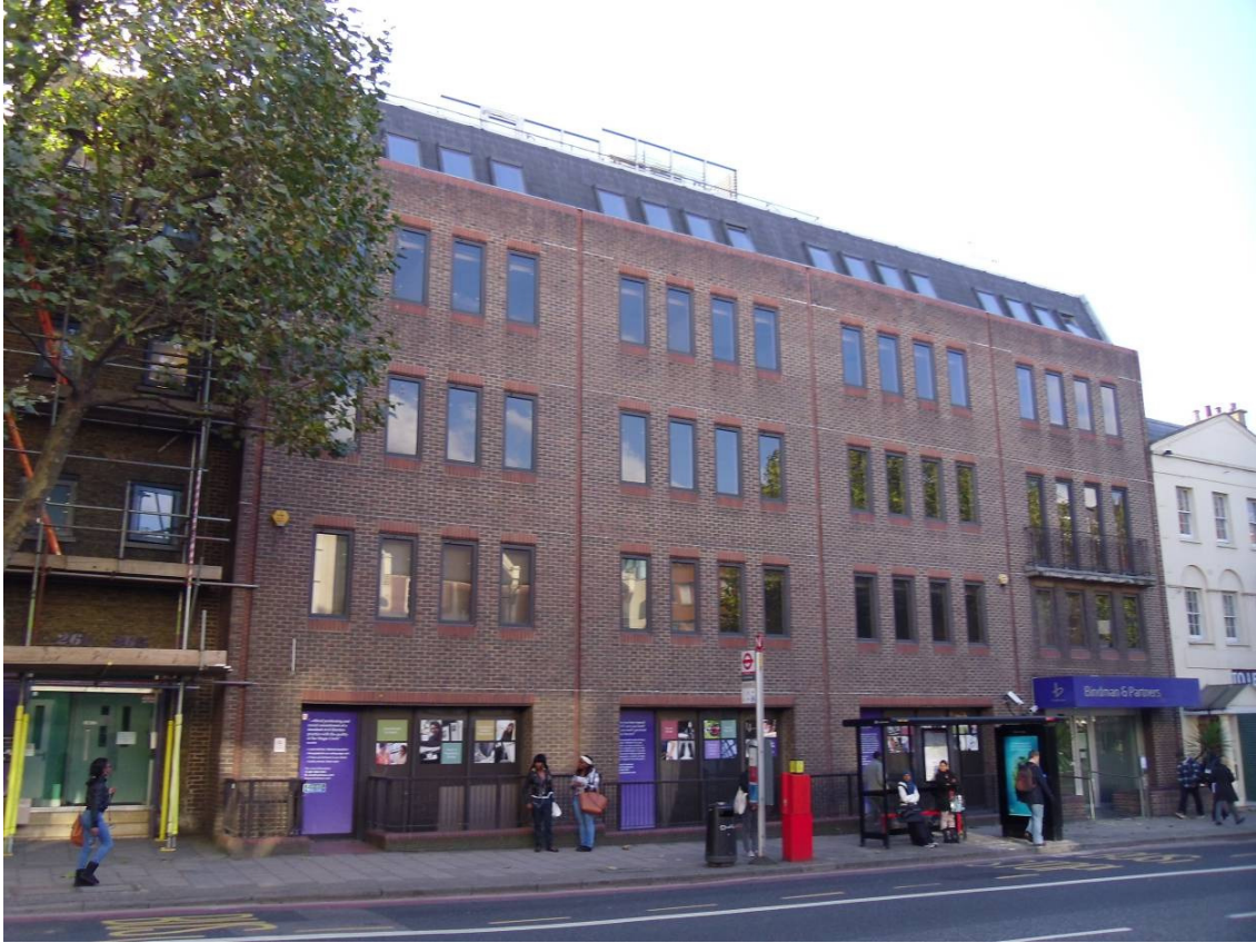
Photo 1.0 showing the existing building at 275 Gray's Inn Road.
