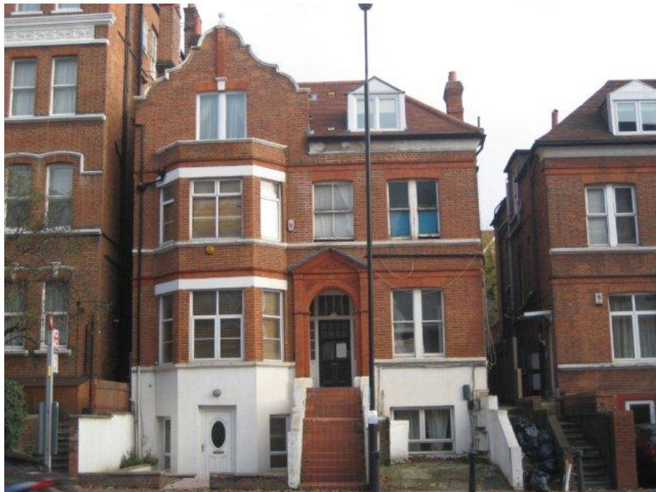
Front elevation of 226 Finchley Road showing existing mixture of timber and uPVC windows
