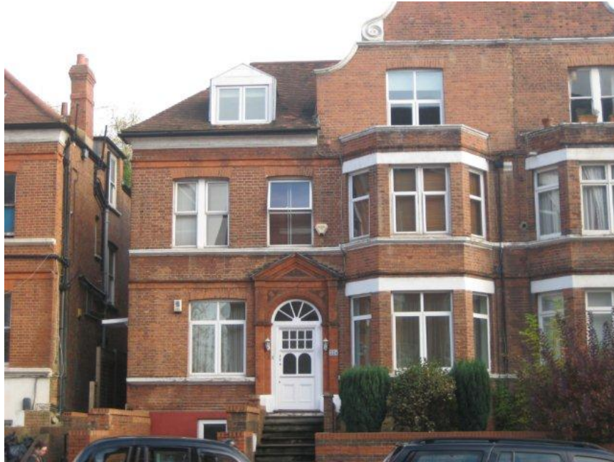
Front elevation of 224 Finchley Road showing existing mixture of styles of uPVC windows
