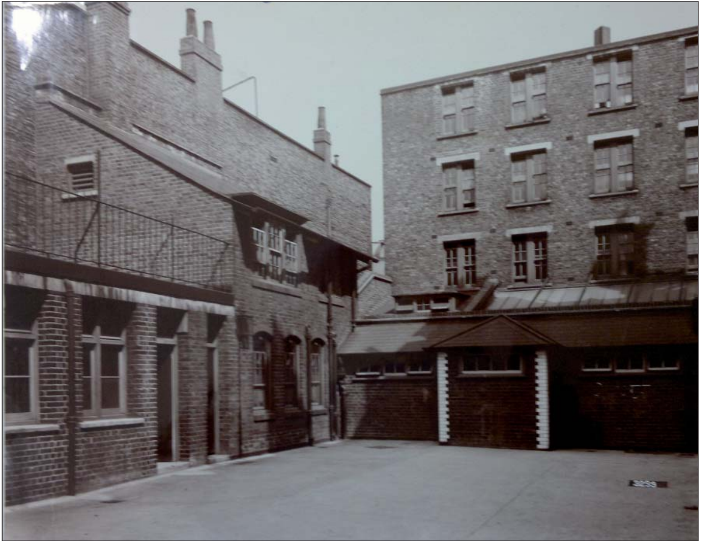
13. Aldwych Workshops with Parker Street House behind 1907 (LMA)
